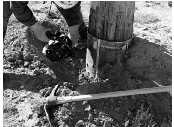
An inspector drills for a core sample on a pole.
