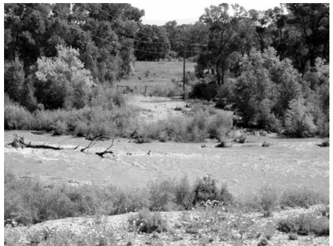
Another pole in danger.
