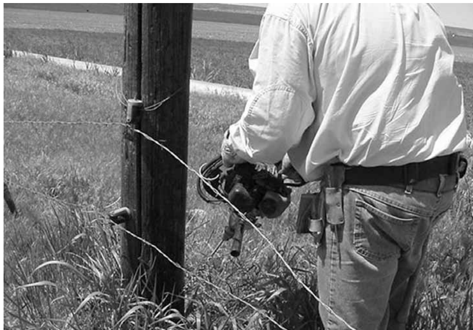
A pole inspector drills for a core sample on a pole.
