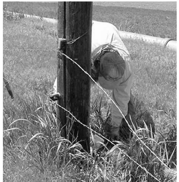
Visual inspection is needed to find damage on the surface of the pole.
